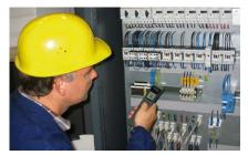
Infrared thermometers are proven time saving tools for predictive maintenance of electrical systems. Check out temperature problems safely with connectors, fuses, electric motors, motor windings, insulations, electrical wiring and electrical cabinets before damages occur.
